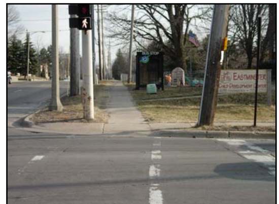
Photo 9: Example of Crosswalk on Corridor
